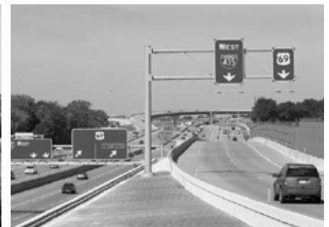
I-435/U.S. 69 INTERCHANGE Overland Park, Kansas
