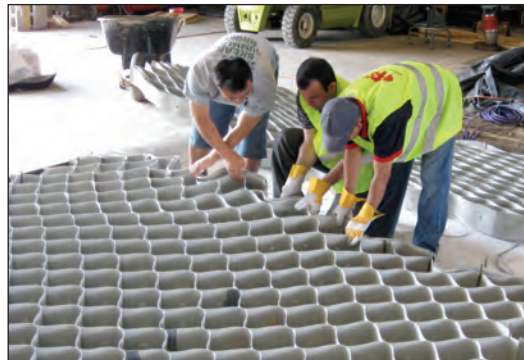
Geocell installation
